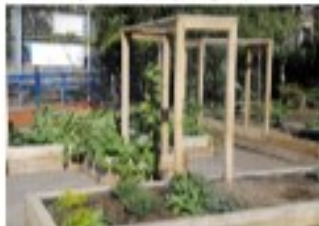
Gourd walk archways constructed from steel mesh and oak and providing green shade for seating in the EP
